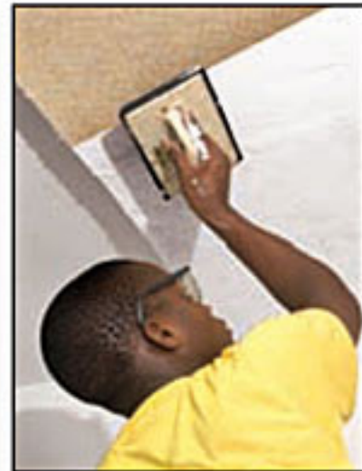
4c) Fit polystyrene cornice to manufacturer's specifications
