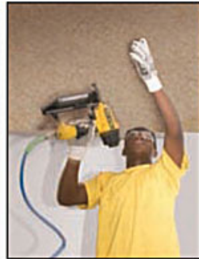
3) Ensure that there is a joint of between 3 -5 mm between edges of boards
