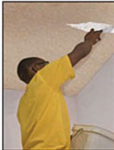
4b) ThermocousteX Plasterboard can be primed with plaster bond and skimmed with either ThermocousteX plaster or 'Creststone'
