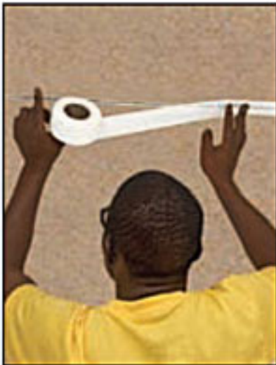
4a) Once installed; - cover strips or joint tape (for skimming) can be used to cover joints and then product is painted or varnished, or;
